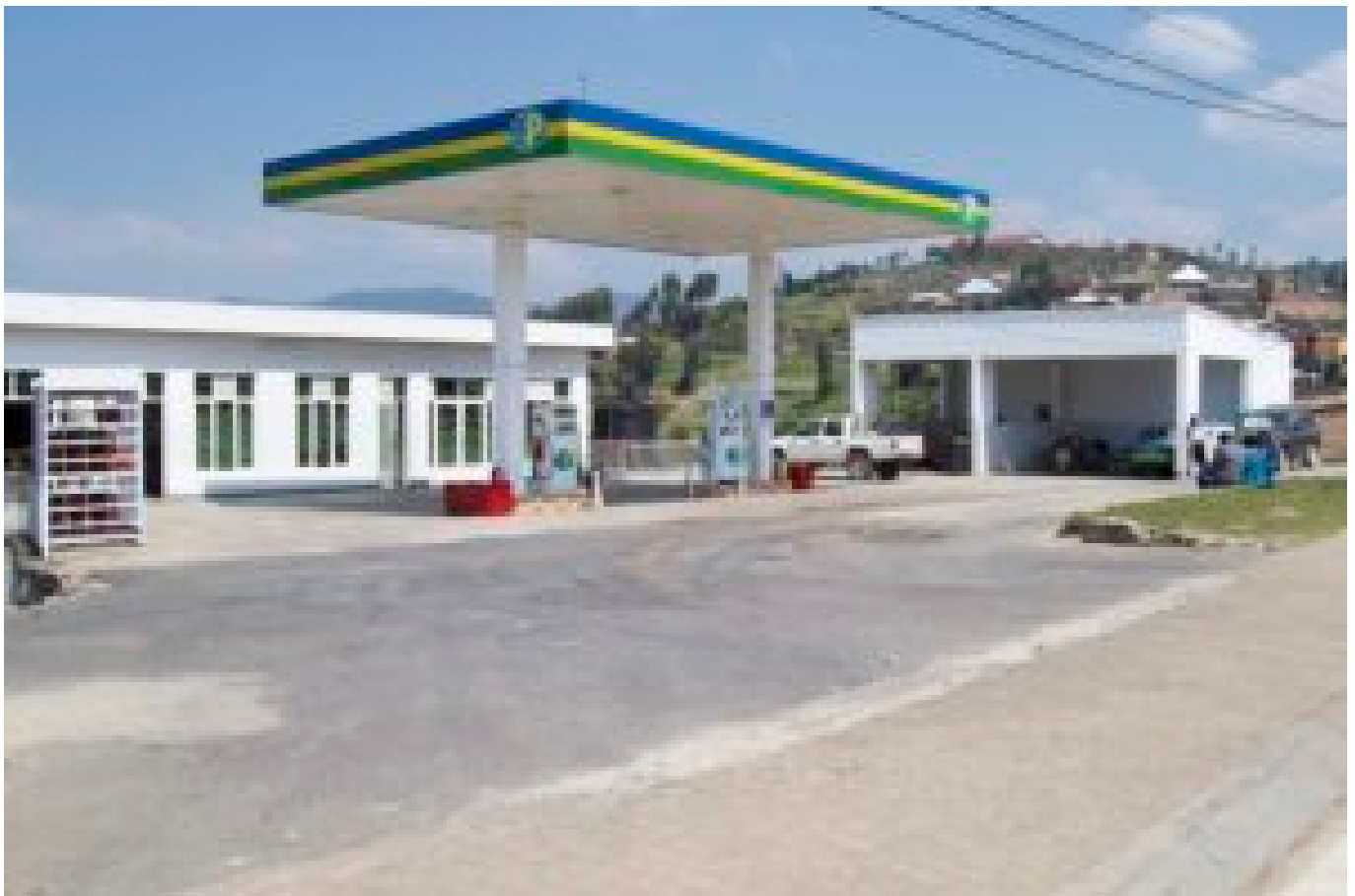
A modern filling gas station in Kitabi built by KOBACYAMU for the neighboring
